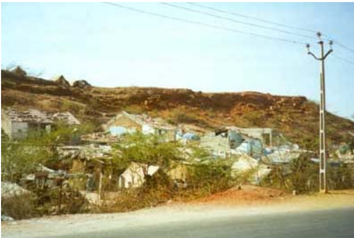
Bhachau Landslide - The land slipped during the 26 th January 2001 earthquake event in Bhachau. Note people are still camped beneath. Monsoon rains could possibly wash the soil downslope.
