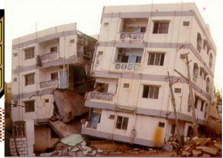
Improperly designed weak or flexible storey leads to poor performance during earthquakes. Many buildings with open ground storeys intended for parking collapsed in the Bhuj earthquake. Seen in the picture is a vertical split of a building due to collapse of a partially open ground storey building. (Source www.nicee.org Earthquake Tips IITK-BMTPC)
