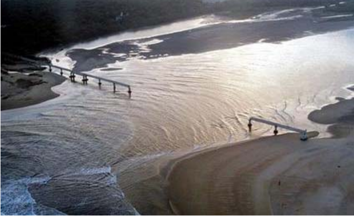
An aerial view of a bridge destroyed by tsunamis near Pondicherry, in the southern Indian state of Tamil Nadu.
