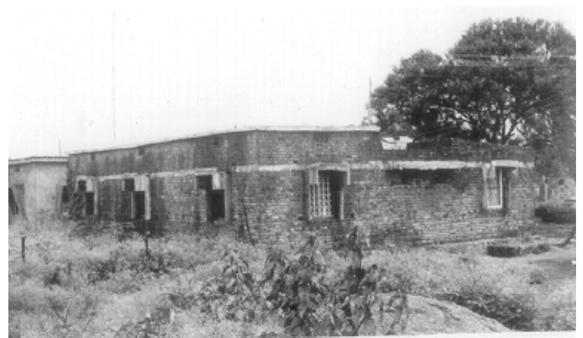
(b) A building with horizontal lintel band in Killari village: no damage
