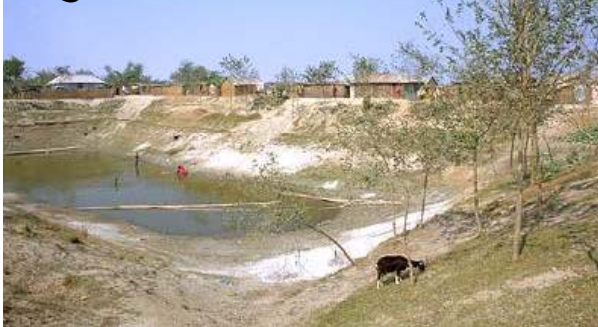
Construction at ground level – risk of inundation
