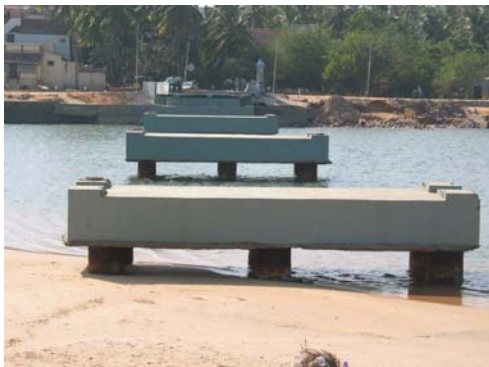
Figure 4.37: Due to tsunami caused by Sumatra earthquake, all the four spans of the deck of this bridge was washed away. One span was moved more than 20 m. Bridge is over the sea and connects Keelamanakudai and Melamanakudai villages in Kanyakumari district in South India.
