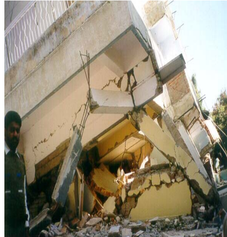
Figure 5.20: Damage to buildings with offsets
