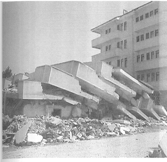
Figure 4.53: Pancaking of a building during the 1999 Izmit earthquake in Turkey
