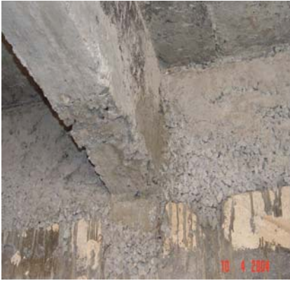
Figure 9.4: Inferior construction
