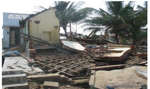
Figure 4.34: Collapse of Adobe houses in a village south of Cuddalore (India) due to tsunami caused by Sumatra earthquake.
