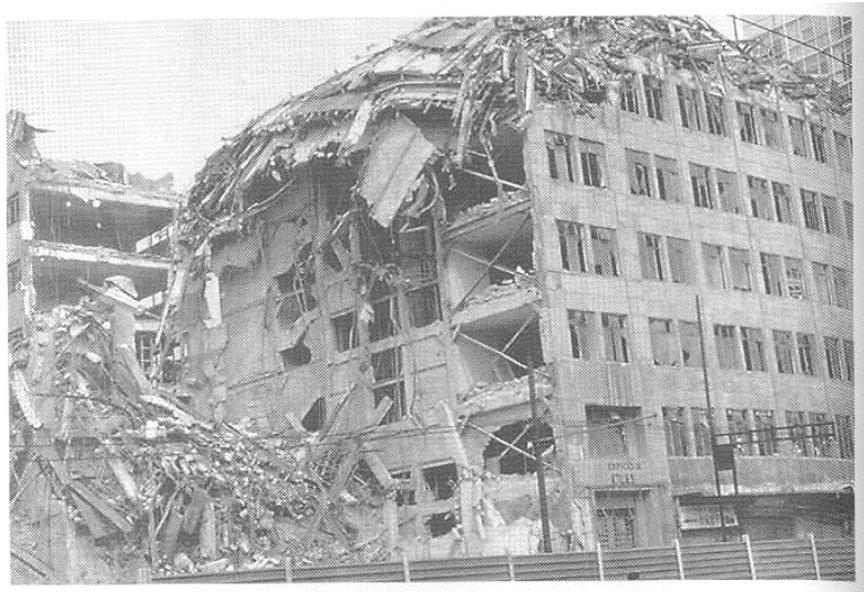
Figure 4.57: Building collapse in Mexico City caused by the 1985 Michoacan earthquake.
