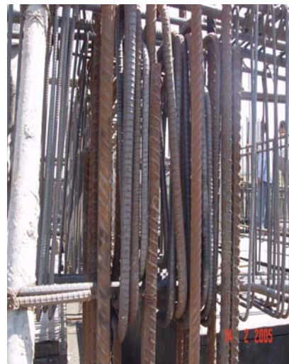
Figure 9.3: Congestion of reinforcement
