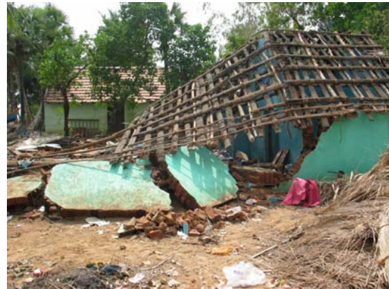
Figure 4.30: Collapse of the adobe houses in Pondicherry (India) due to tsunami caused by December 26, 2004 Sumatra earthquake.
