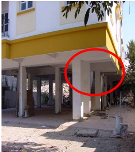
Figure 5.20: Damage to buildings with offsets
