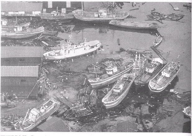
Figure 4.28: Tsunami damage caused by the 1964 Niigata earthquake in Japan.
