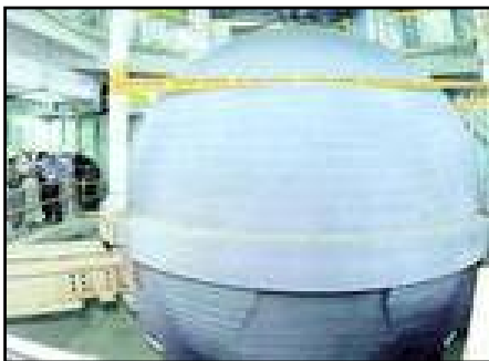
Figure 12.50: Ball shaped damper in the Taipei 101, Taiwan
