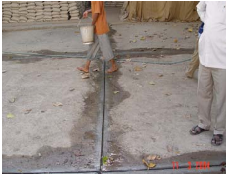
Figure 9.6: Improper gaps
