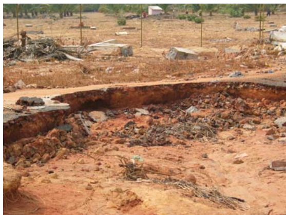
Figure 4.31: Erosion of a pakka road in Pondicherry (India) due to tsunami caused by Sumatra EQ.
