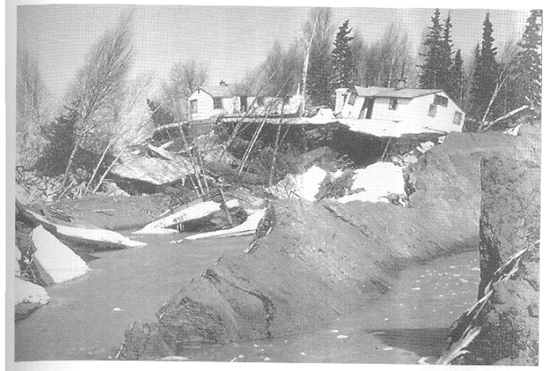
Figure 4.25: Damage caused by movement of the Turnagain Heights landslide during the Alaskan EQ.
