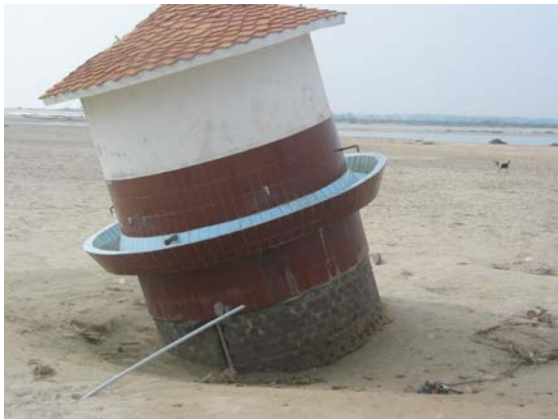
Figure 4.33: Damage to a structure used for drinking water near Cuddalore (India) due to settlement of soil caused by tsunami generated by Sumatra EQ.
