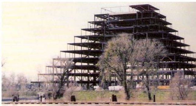
Figure 12.18: View of onsite construction
