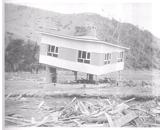
Figure 4.29: Tsunami damage caused by the 1970 Chile earthquake.
