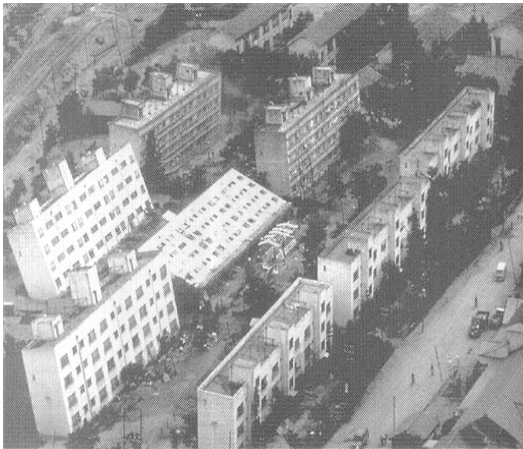
Figure 4.7: Kawagichi-cho apartment buildings suffered liquefaction-induced bearing capacity failure during the Niigata (Japan) earthquake on June 16, 1964.
