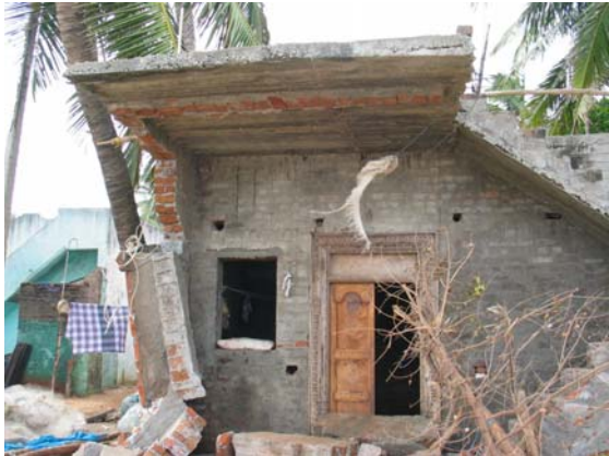
Figure 4.32: Damage to brick masonry construction in Cuddalore (India) due to tsunami caused by Sumatra EQ.
