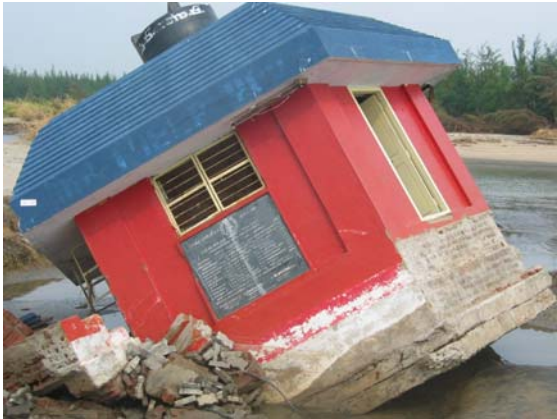
Figure 4.35: Damage to a police check post due to settlement of soil below at Nagapattinam beach (India) due to tsunami caused by Sumatra earthquake.
