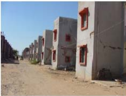
Figure 4.58: Pink sandstone up to 600 mm in size was used for 2-story houses
