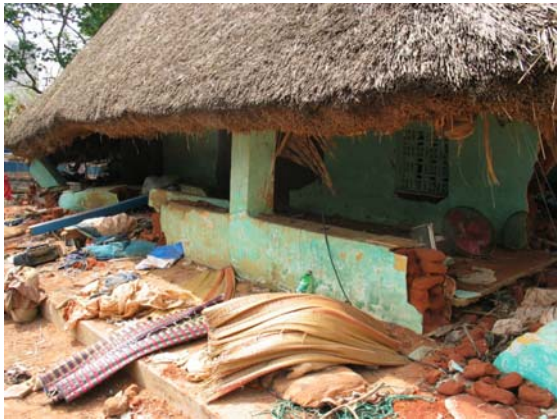
Figure 4.30: Collapse of the adobe houses in Pondicherry (India) due to tsunami caused by December 26, 2004 Sumatra earthquake.
