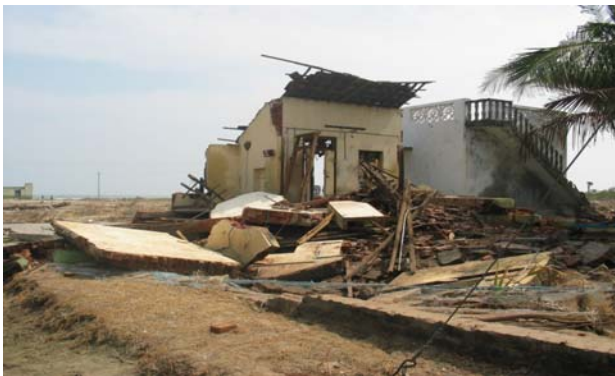
Figure 4.34: Collapse of Adobe houses in a village south of Cuddalore (India) due to tsunami caused by Sumatra earthquake.
