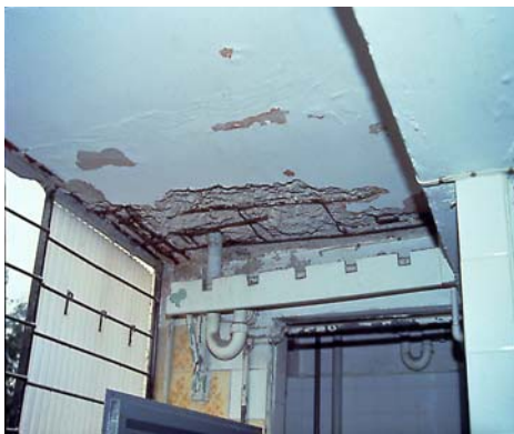
Figure 9.8: Leaking Toilets
