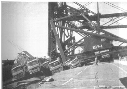
Figure 4.13: Collapse of a crane due to about 2 m of lateral movement of the retaining wall of Rokko Island during the Kobe earthquake.
