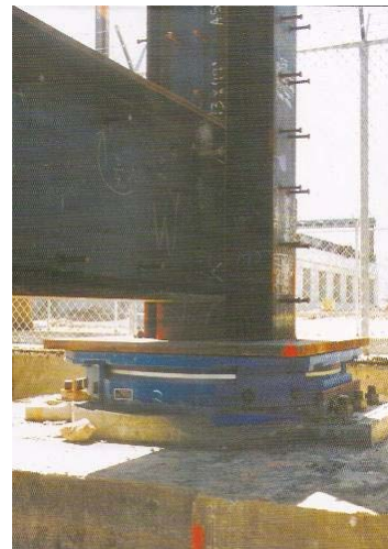
Figure 12.37: Detail of Friction Pendulum Bearing Isolator
