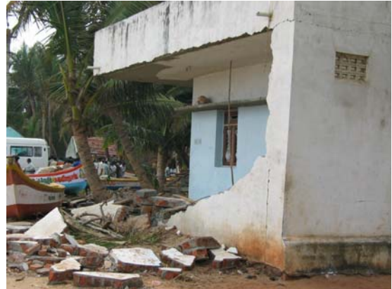
Figure 4.32: Damage to brick masonry construction in Cuddalore (India) due to tsunami caused by Sumatra EQ.
