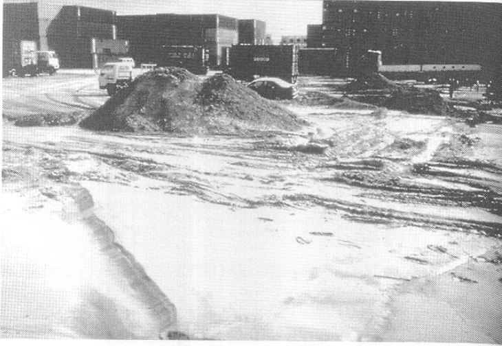
Figure 4.10: The interiors of Rokko and Port islands settled as much as 1 m with an average of about 0.5 m due to liquefaction caused by the Kobe earthquake. This liquefaction-induced settlement was accompanied by the eruption of large sand boils that flooded many areas and covered much of the island with sand boil deposits. In this photograph, a stockpile has been created out of this sand.
