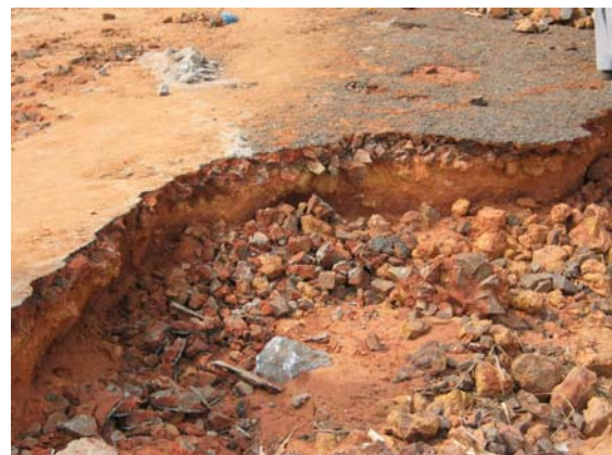
Figure 4.31: Erosion of a pakka road in Pondicherry (India) due to tsunami caused by Sumatra EQ.
