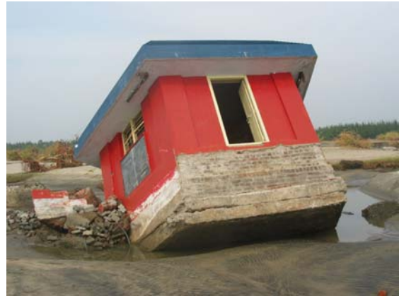
Figure 4.35: Damage to a police check post due to settlement of soil below at Nagapattinam beach (India) due to tsunami caused by Sumatra earthquake.
