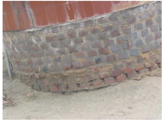
Figure 4.33: Damage to a structure used for drinking water near Cuddalore (India) due to settlement of soil caused by tsunami generated by Sumatra EQ.
