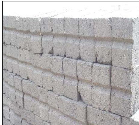
Figure 9.16: Poor workmanship
